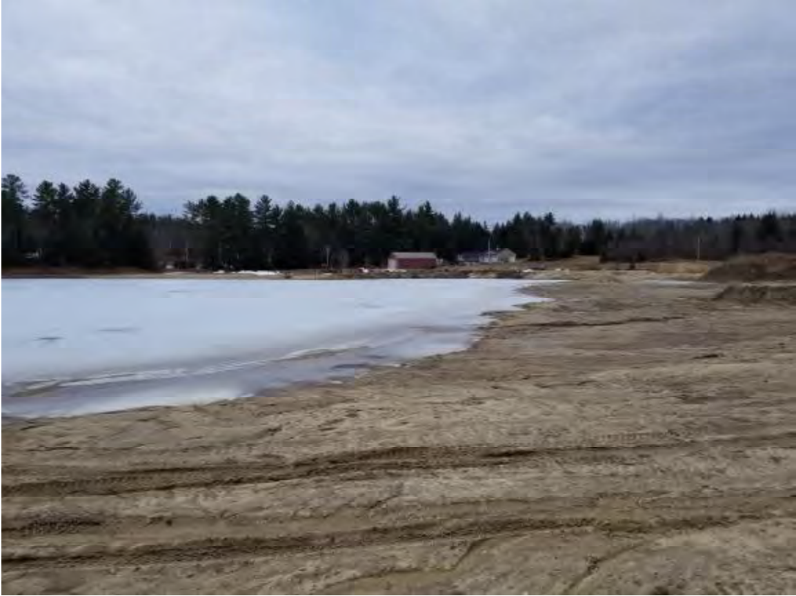
Photo 3: View to north/northwest of active excavation.
