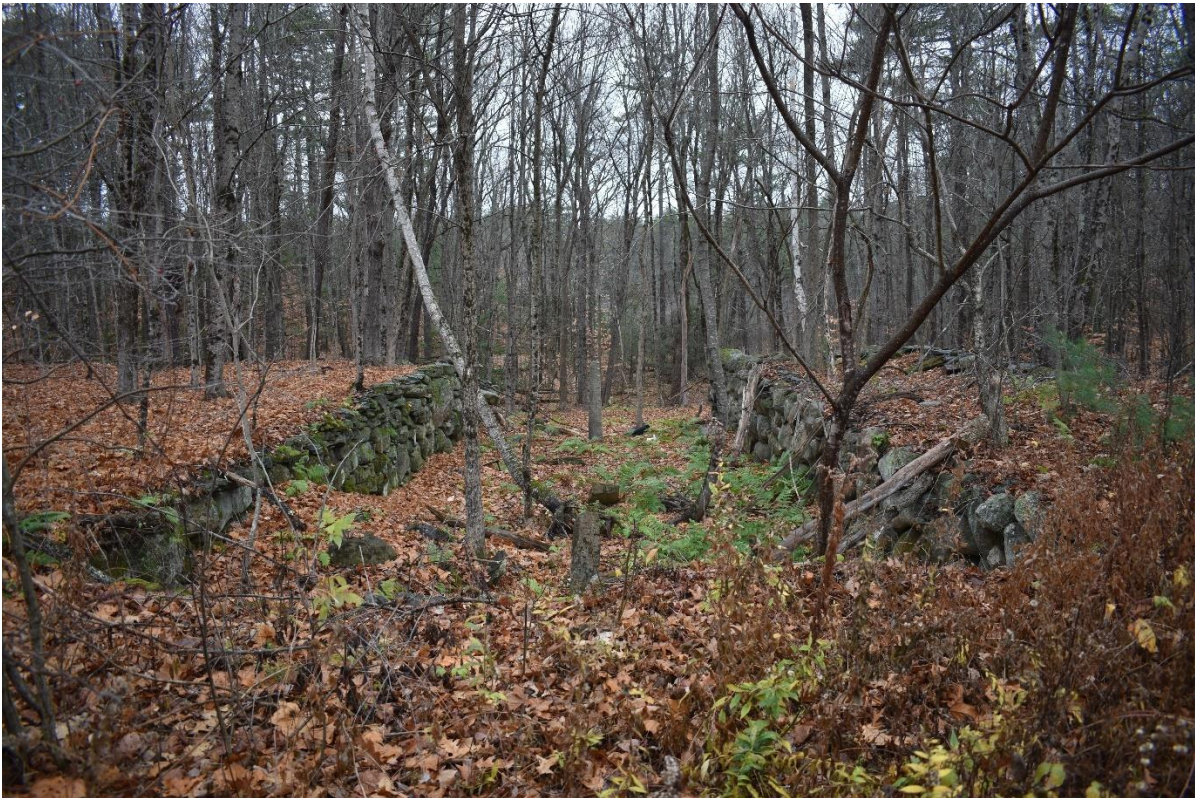
Plate 3. The Nealley-Gile barn foundation, view west.
