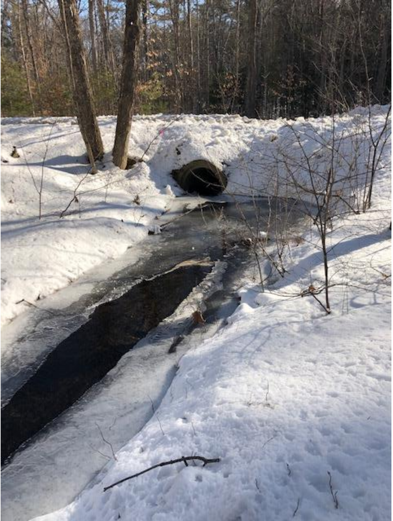
10. Culvert at inlet under Poor Farm Road.
