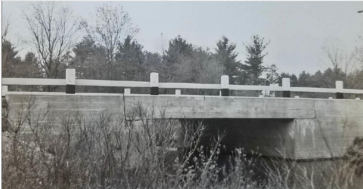
FIGURE 10: Photo of Nottingham Bridge 141/127 on bridge card dated May 7, 1941, showing east elevation before 1970 widening.
