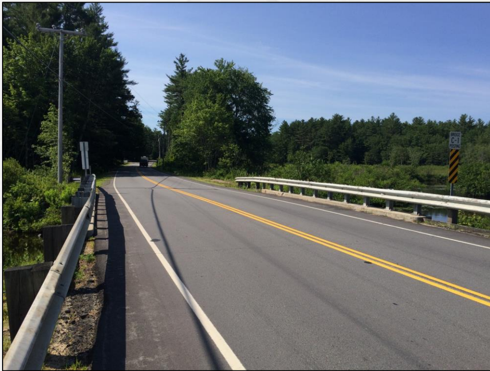
Looking South Along NH Rt.152
