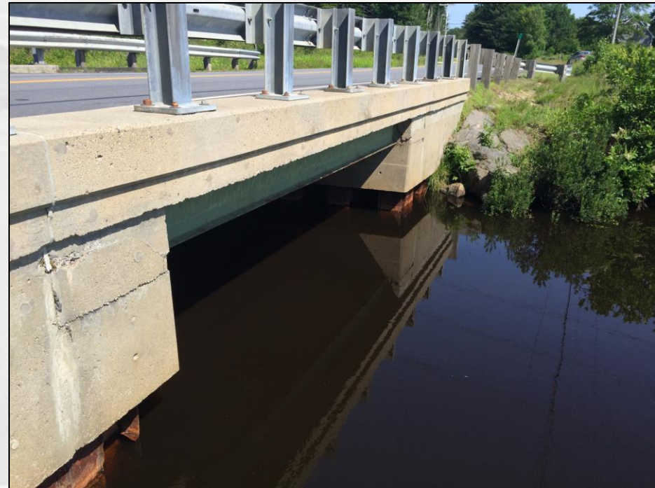
Bridge Upstream Elevation
