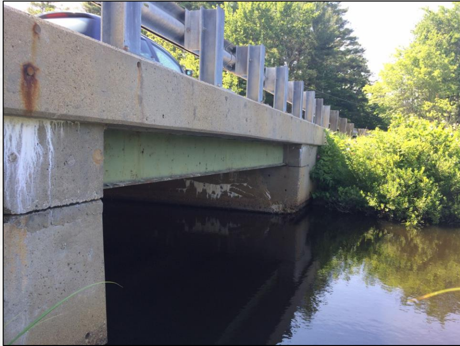
Bridge Downstream Elevation
