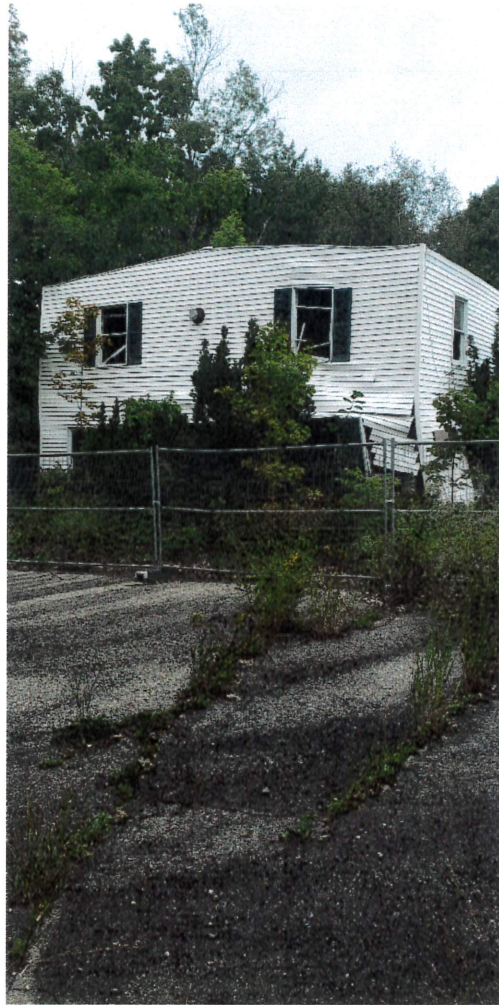
BUILDING #1 WOOD STRUCTURE AND SECURITY FENCE (#2)
