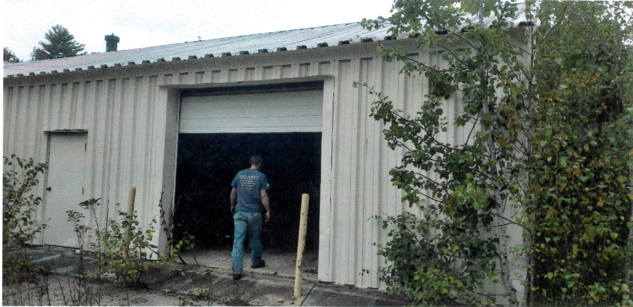
BUILDING #2 OVERHEAD DOOR (#4)
