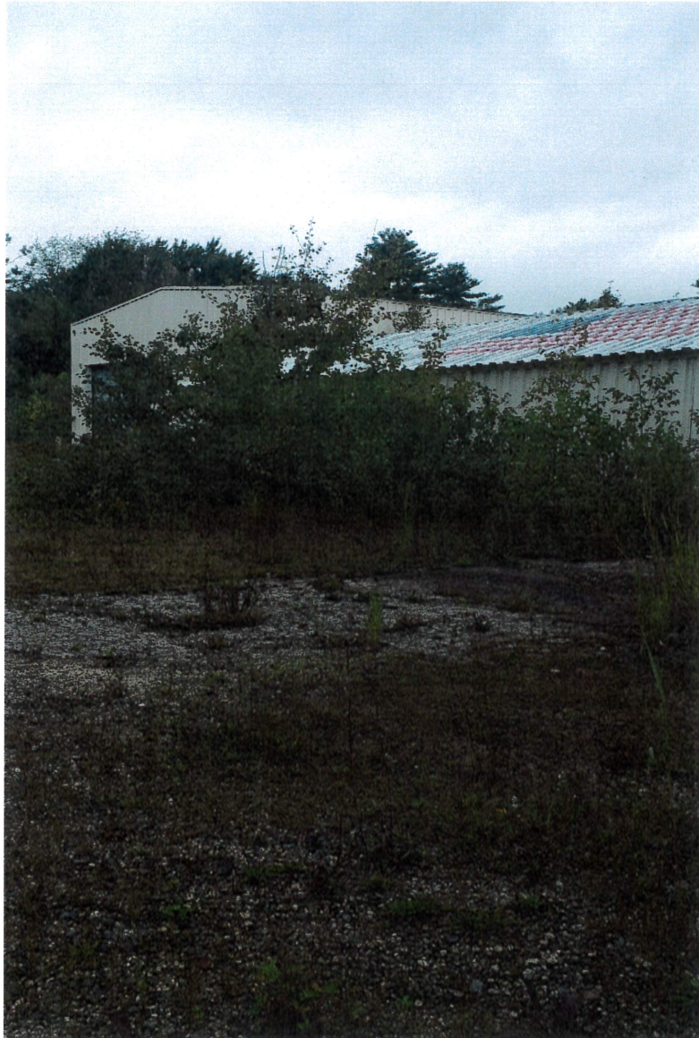
BUILDING #2 & 3 LOOKING NORTHWEST (#3)
