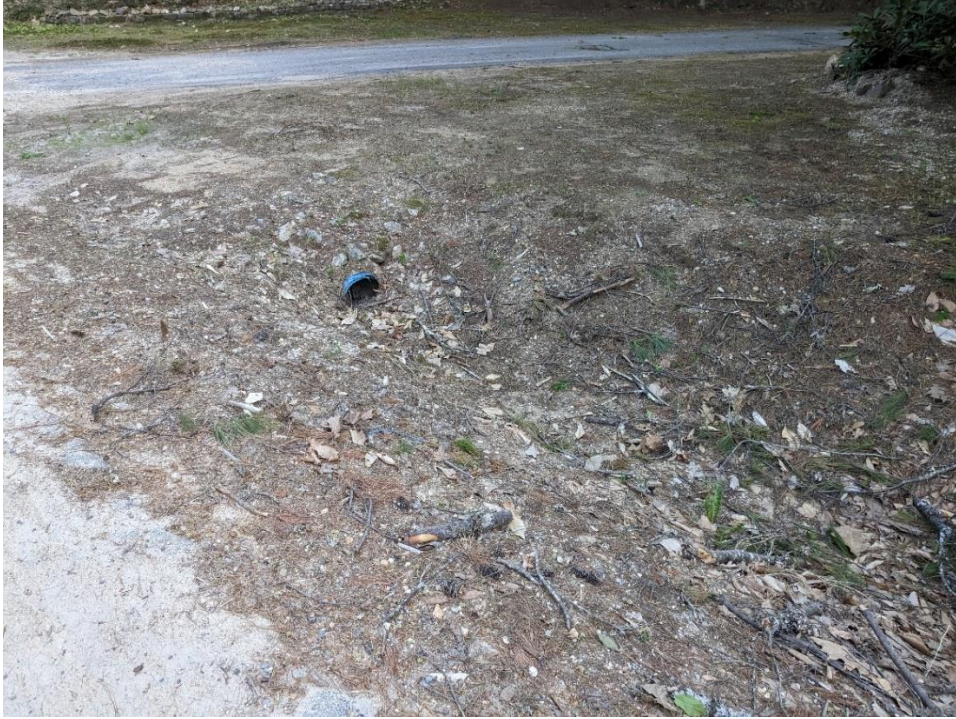
6. Culvert next to Weston driveway off Fort Hill Rd.
