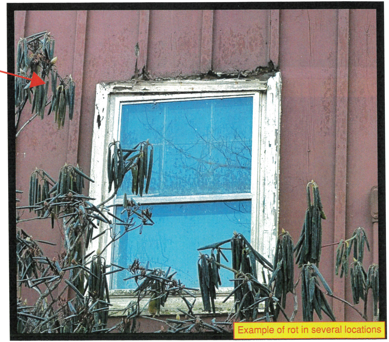
Example of rot and rodent/bird damage in several locations
