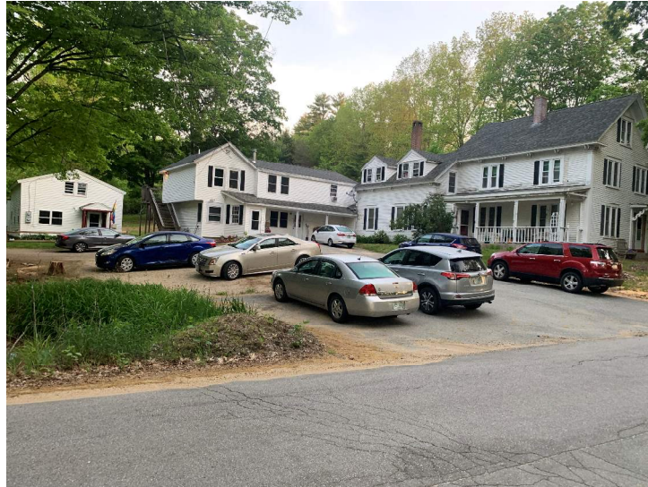
Figure 4 Unpermitted Overflowing Parking
