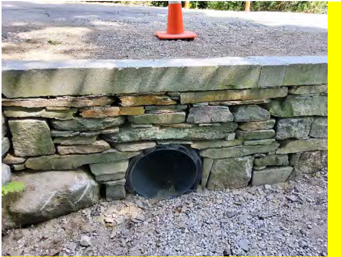
Headwall work on Flutter Street
