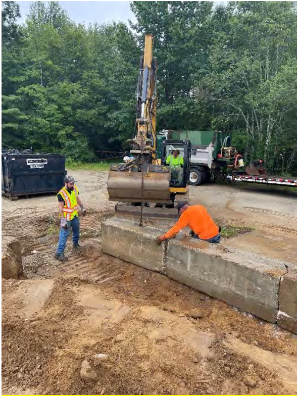
Recycling center retaining wall repairs
